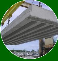
Precast elements Precast pre-stressed roof elements & beams, façade panels, tanks, containers, pipes, piles, etc.
